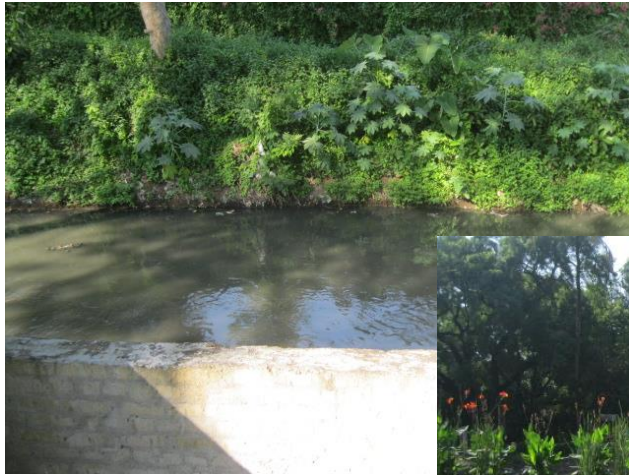
Raw sewage in nallah
